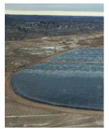
**Final Cover System.** An impermeable "cover" is placed over waste to prevent air and water from getting into the landfill mass.
